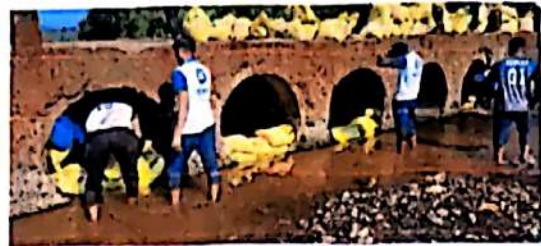
Constructed Vanrai Bandhara on Arjuna river
